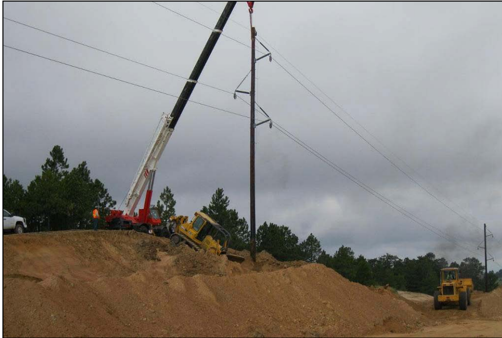
Hodgen Road (Phase 2): Slope Grading and Tri-State Pole Adjustment
