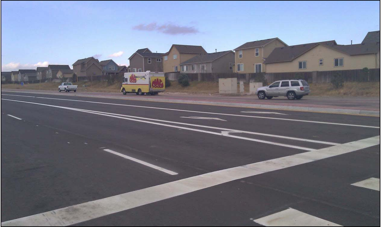
Meridian Road (North): Completed concrete median, paving and striping at the intersection of Meridian Road and Woodmen Road.
