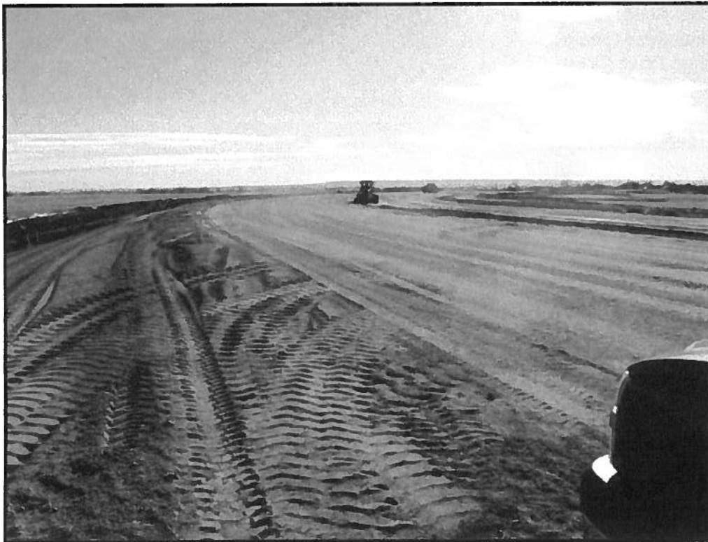
Grading Road Platform at Stapleton Road (West)
