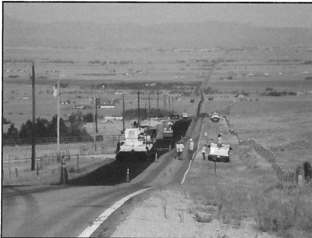
Asphalt Overlay on Judge Orr Road
