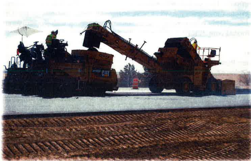
Marksheffel Road South Paving
