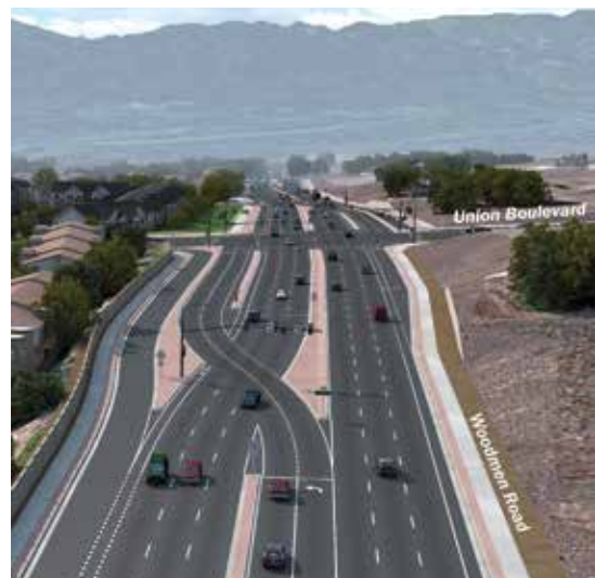
A rendering of the Continuous Flow Intersection planned for Woodmen Road and Union Boulevard
