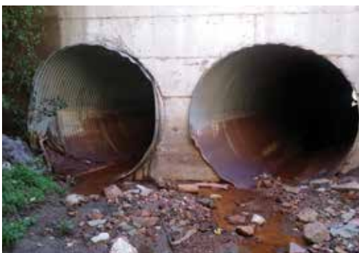
Much of the corrugated metal pipe used in constructing our bridges is nearing the end of its service life.
