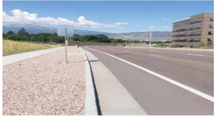
Three key segments of Austin Bluffs parkway were widened from four lanes to six.
