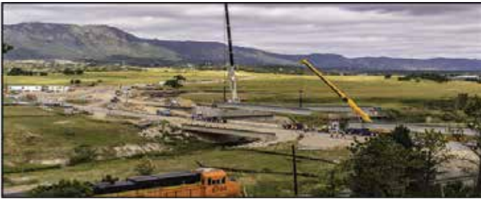
Girder erection for Baptist West bridge
