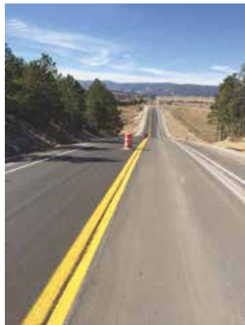
County Line Road, looking west
