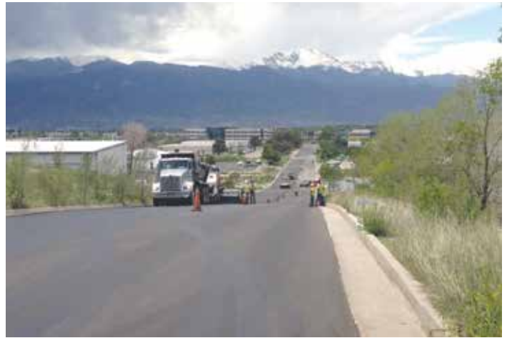
Paving operation on Terminal Avenue
