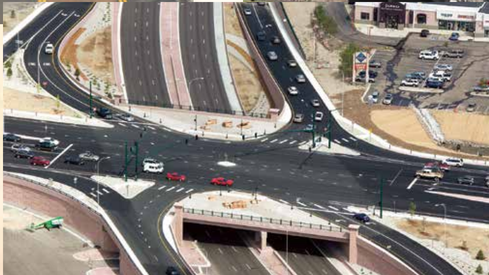
Cover photo: Newly completed three-span Baptist Road bridge over Monument Creek and railroad tracks
