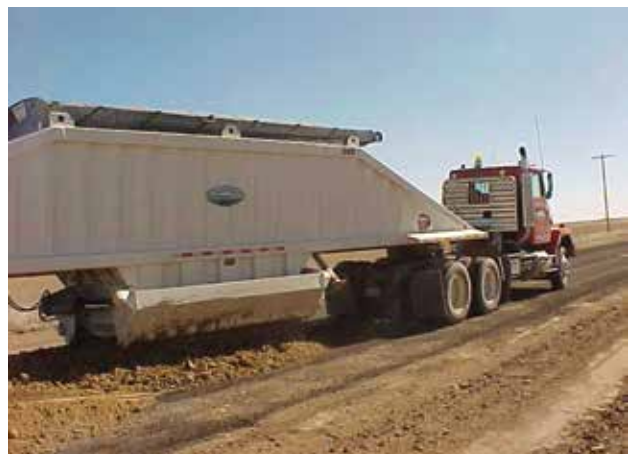
Graveling on Scott Road
