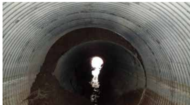
Much of the corrugated metal pipe used in constructing our bridges is nearing the end of its service life.
