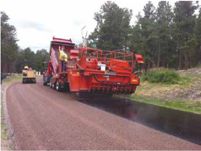
Applying chip seal
