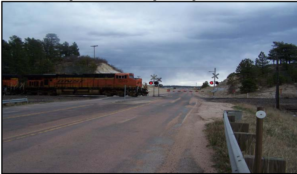
Baptist Road – Existing at-grade RR crossing
