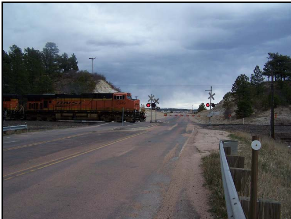
Baptist Road – Existing at-grade RR crossing
