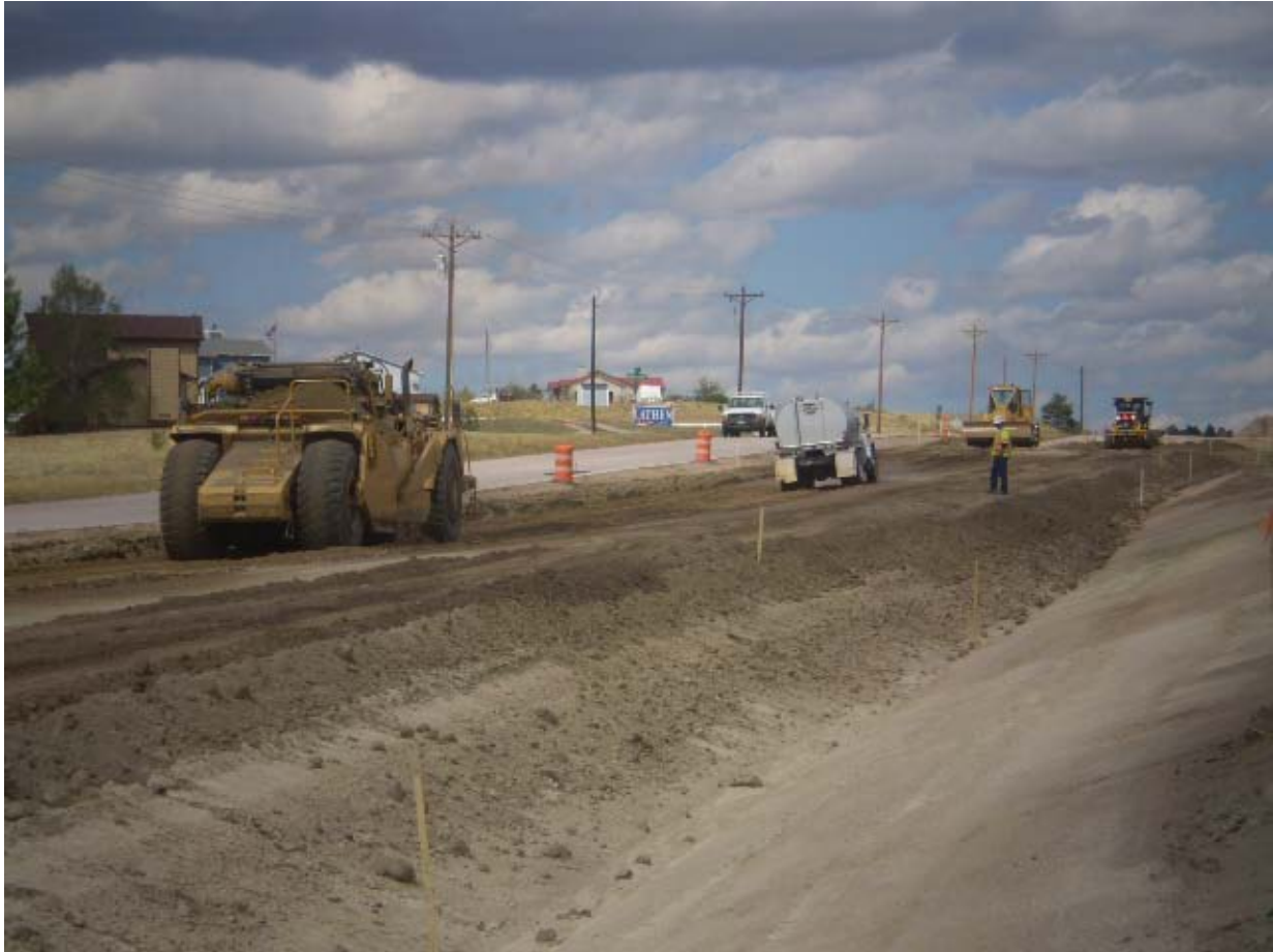
Meridian Road (North) Phase 2: Earthwork of new Northbound lanes
