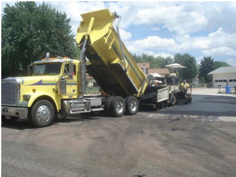
Paving operation on Harvard Street cul-de-sac
