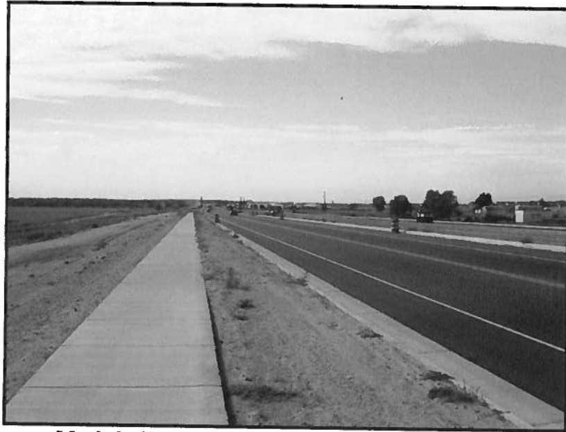
Marksheffel Road (North): new north bound lanes between Constitution and North Carefree
