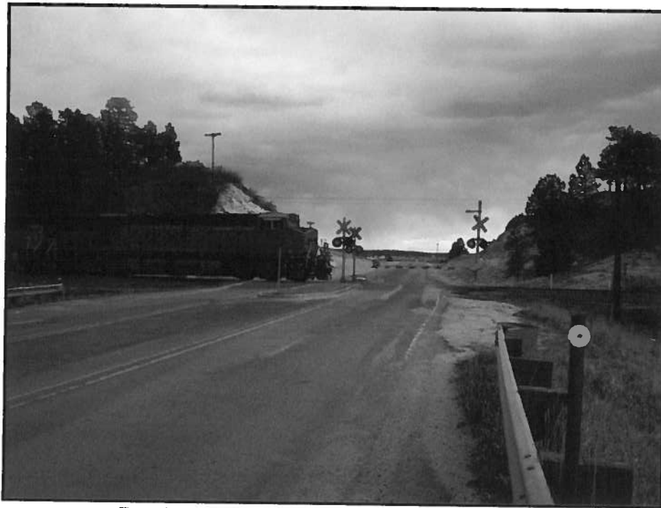
Baptist Road – Existing at-grade RR crossing
