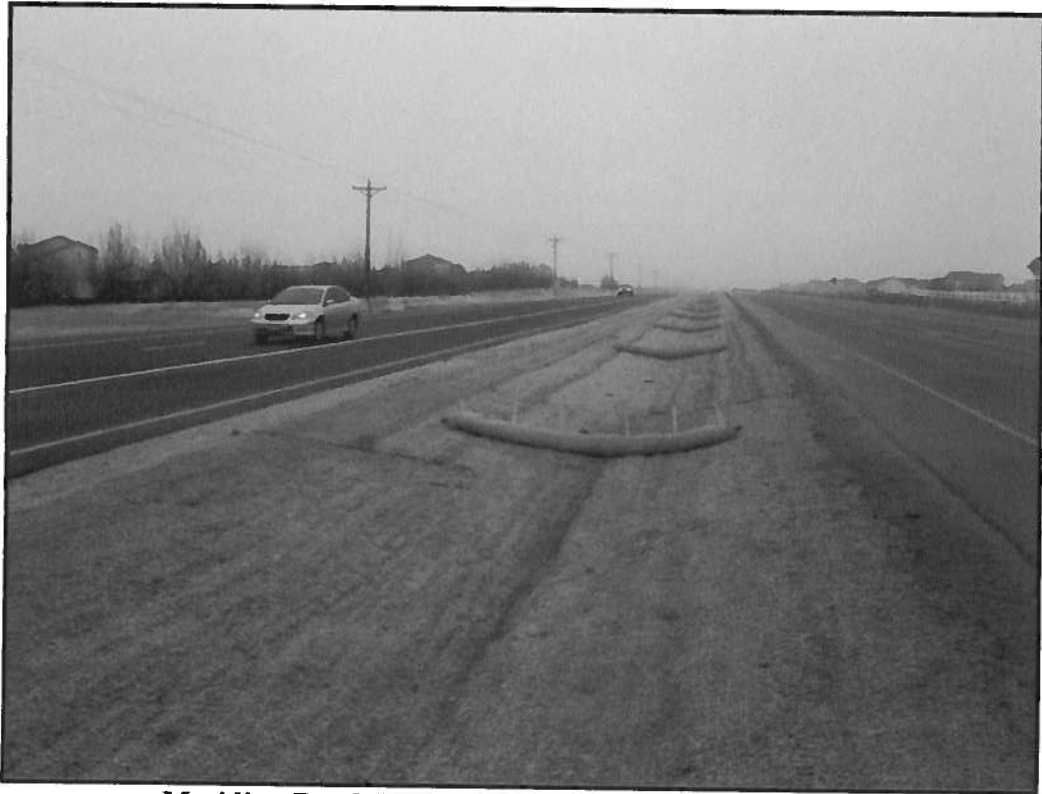
Meridian Road (North): Completed southbound lanes
