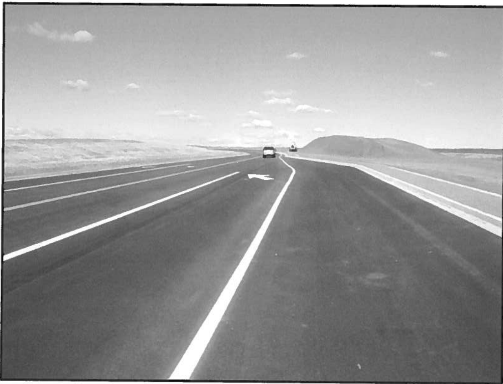
Stapleton Road (West): completed paving and striping
