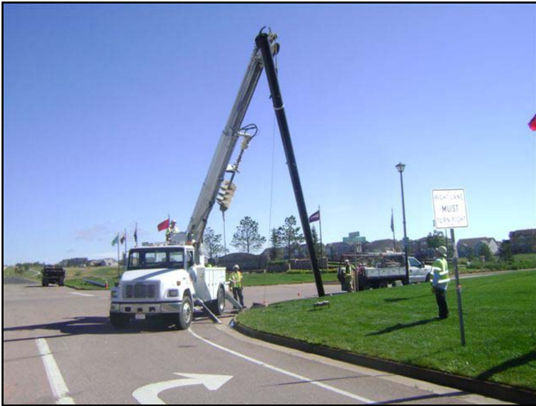
Meridian (North) Project: Signal installation at Londonderry Drive/Meridian Road
