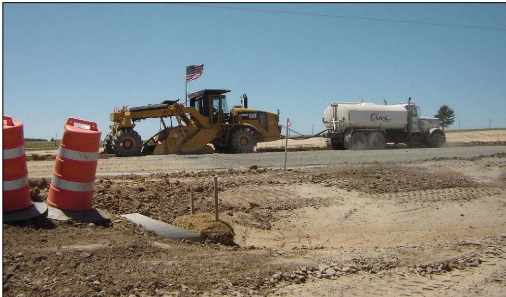
Hodgen Road (Phase 2): Mainline Soil Cement Treatment
