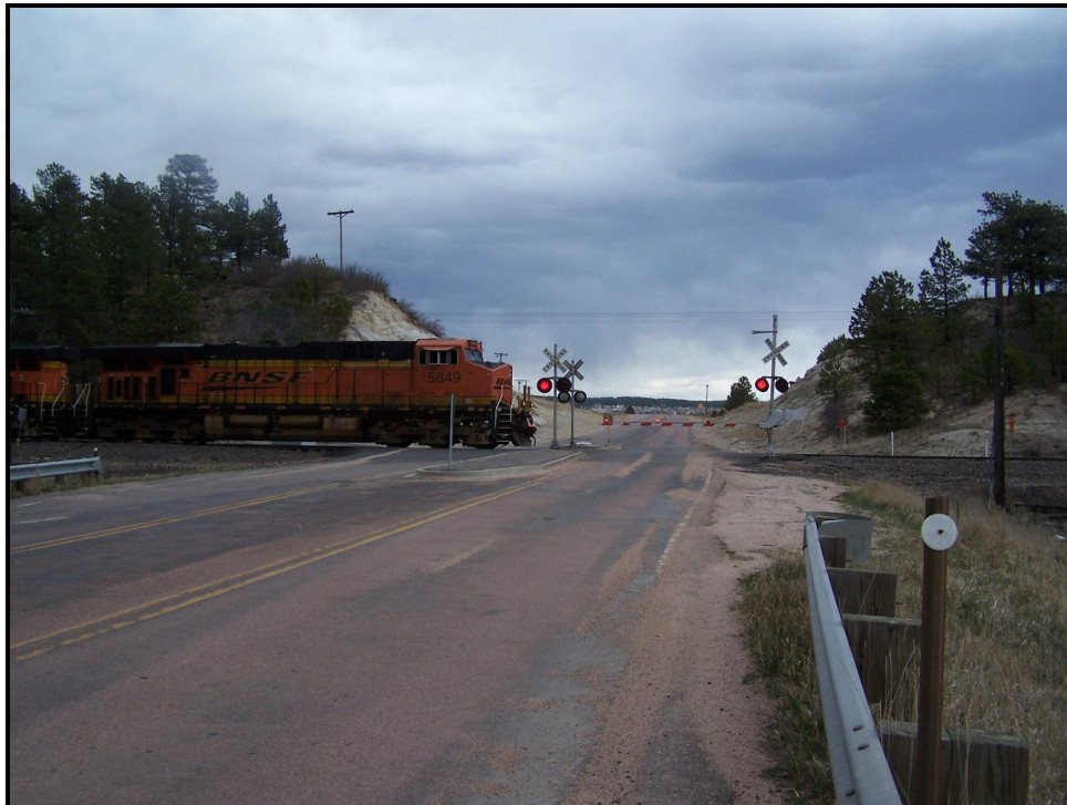
Baptist Road – Existing at-grade RR crossing
