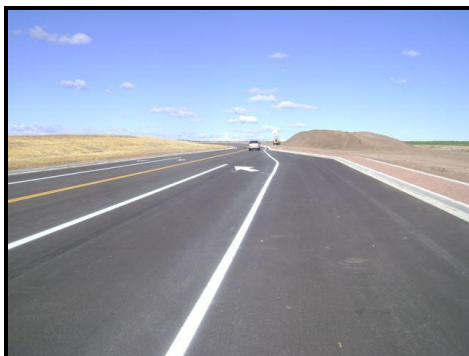
Stapleton Road (West): completed paving and striping.
