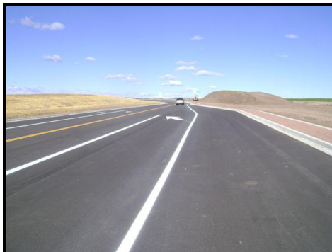
Stapleton Road (West): completed paving and striping.
