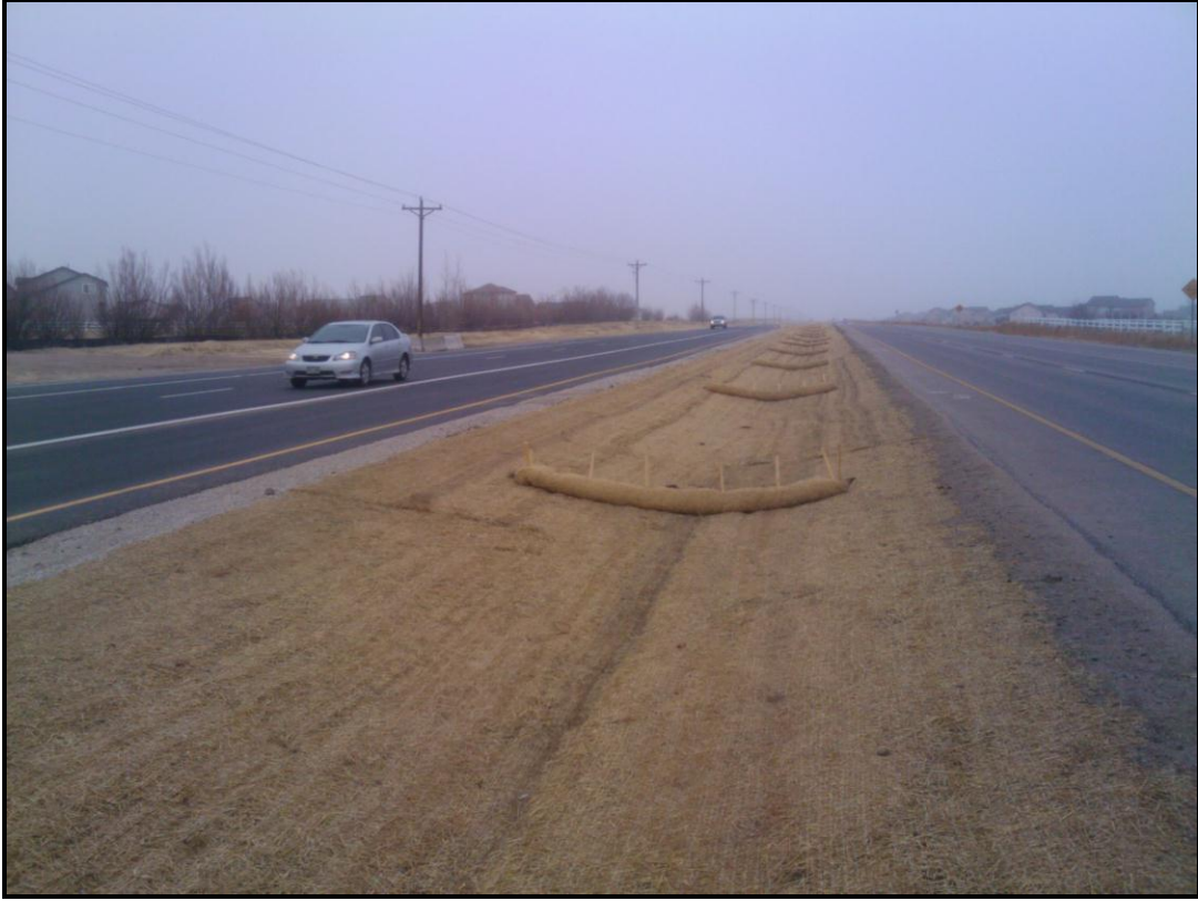
Meridian Road (North): Completed southbound lanes
