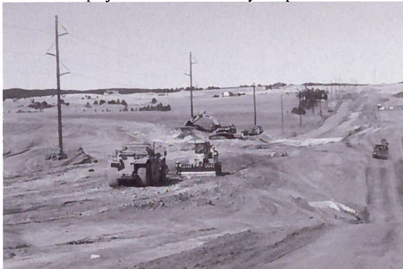
Roadway Construction looking west along Hodgen Road
