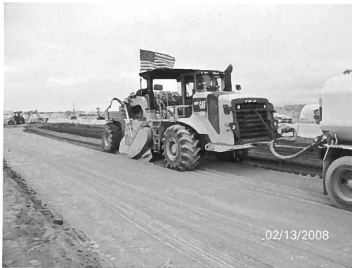
Subgrade Stabilization
