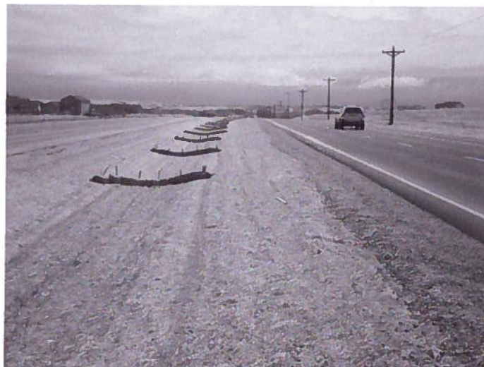
New Southbound lanes looking South
